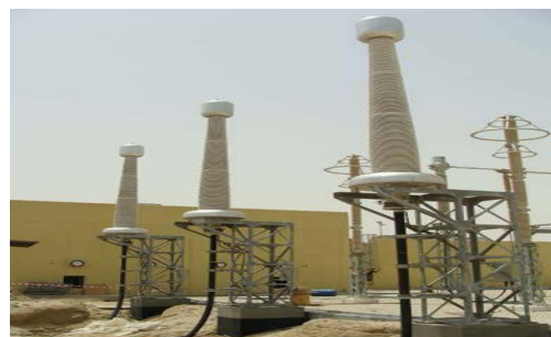
Figure 6: 400 kV Termination under construction
